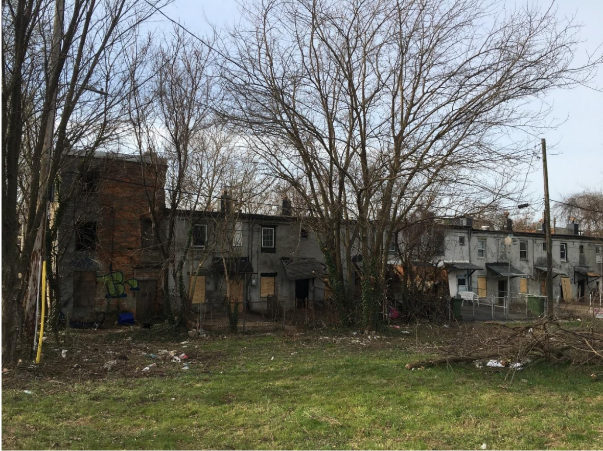
Figure 8: 1102-1118 Sarah Ann Street rear facades.
