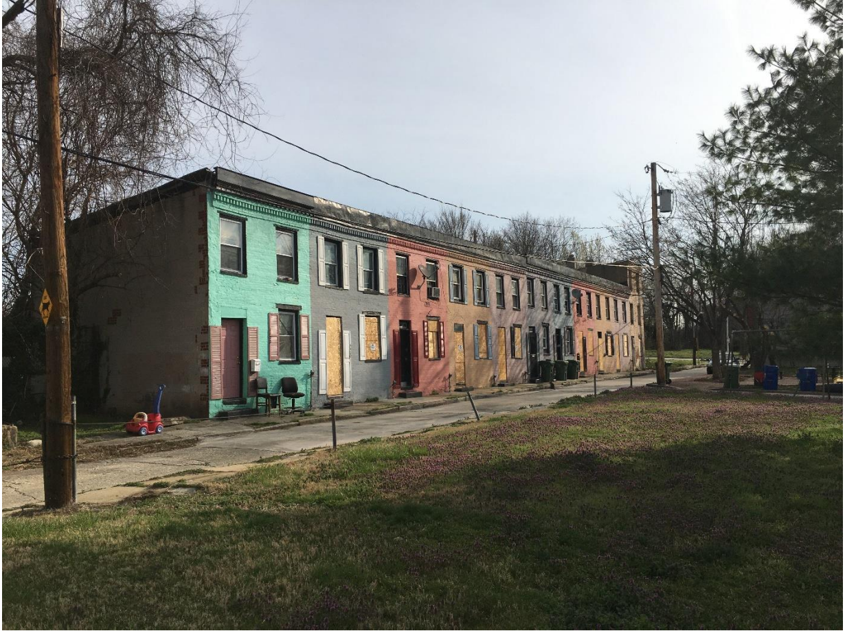
Figure 1: 1124 (vacant lot) through 1102 Sarah Ann Street. These buildings are currently owned and maintained by HCD.
